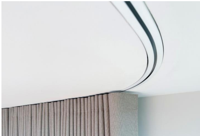
Trackrim Click Curved Section finished installation.
