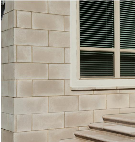
Extra care should be taken to avoid mortar droppings and smears as modified mortar is difficult to remove. Be prepared to clean the stone immediately before the mortar has time to set. Do not use acidic cleaners. Consult the modified mortar manufacturer for additional cleaning information.
