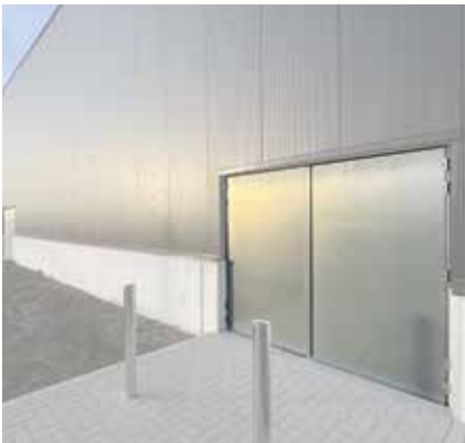
Emergency exit / Exterior
