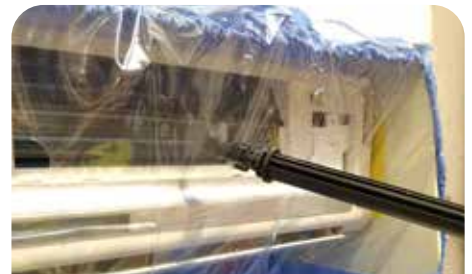
Battery cleaning through cleaning machine hole
