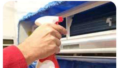
Battery cleaning without protective cover
