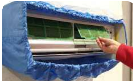
Removing the filters
