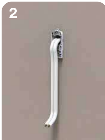
2 Insert the refrigeration lines and the power cable into the wall hole
