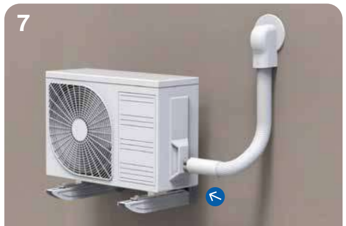
7 Flare the refrigerant pipes and fix them to the taps of the outdoor unit, connect the power supply. Approach and position the rubber sleeve near the taps
