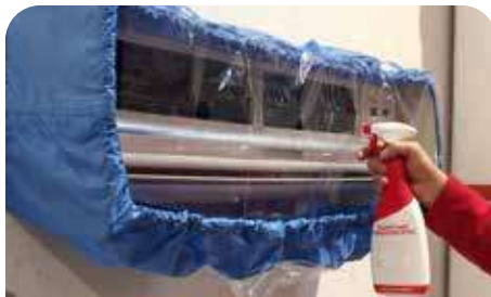
Battery cleaning with protective cover
