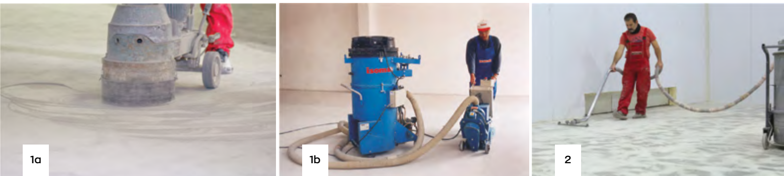
1a. Treating the surface with a terrazzo polishing machine. 1b. Grinding the surface by shot blasting. 2. Treatment residue and dust are cleaned with a high-suction vacuum cleaner.
