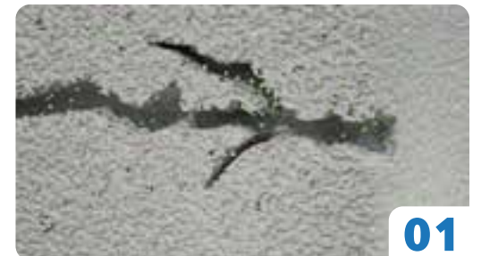
Typical leaking crack in concrete.
