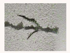
**02** As moisture appears, AQUAMAT-ADMIX, calcium hydroxide and other by-products of cement hydration dissolve in the capillary water.
