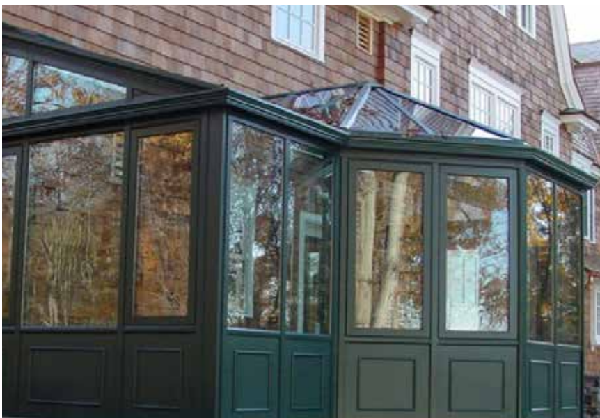
RESIDENCE | REDDING, CT Straight Eave Lean-To Conservatory with Irregular Conservatory Nose Dormer
