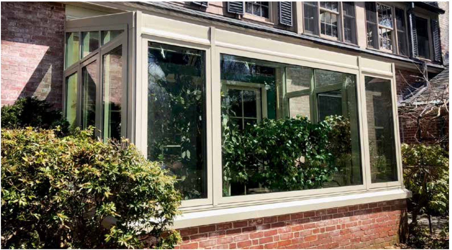
RESIDENCE | ANDOVER, MA Straight Eave Lean-To Sunroom
