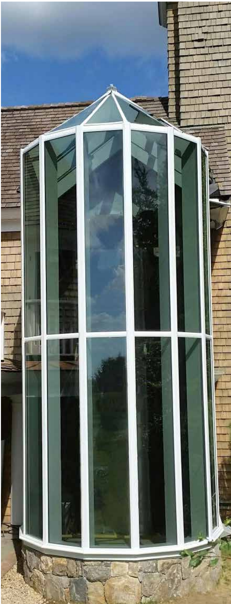
RESIDENCE | NORTH SALEM, NY 17-Sided Conservatory Nose
