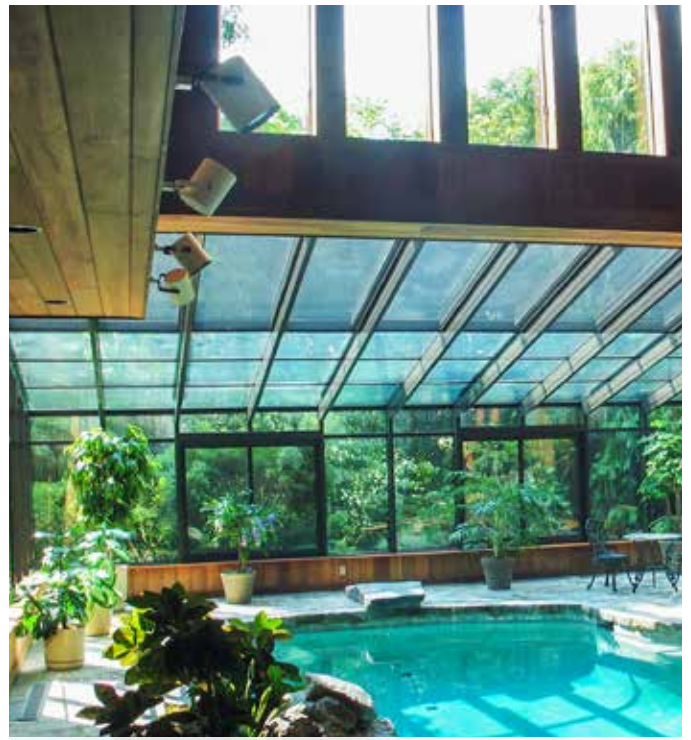
RESIDENCE | STRATFORD, CT Straight Eave Lean-To Retractable Skylight
