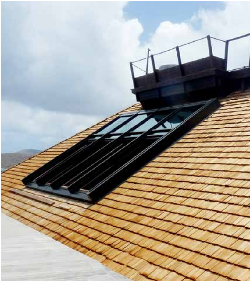
NECKER ISLAND HOTEL | BRITISH VIRGIN ISLANDS Single Slope Retractable Skylight
