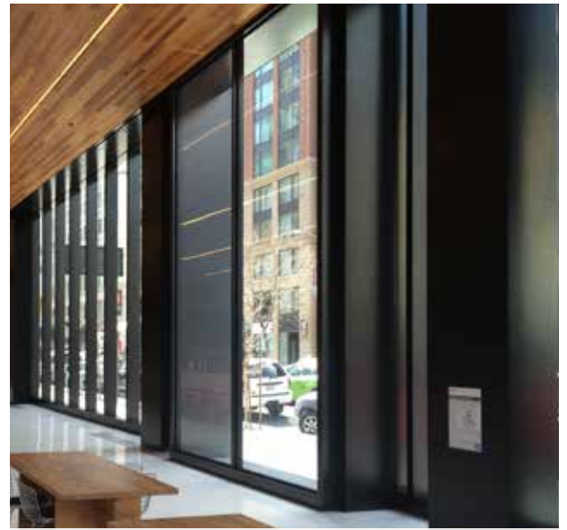
LINKEDIN HEADQUARTERS | SAN FRANCISCO, CA 20ft Motorized Dual Track Sliding Glass Doors
