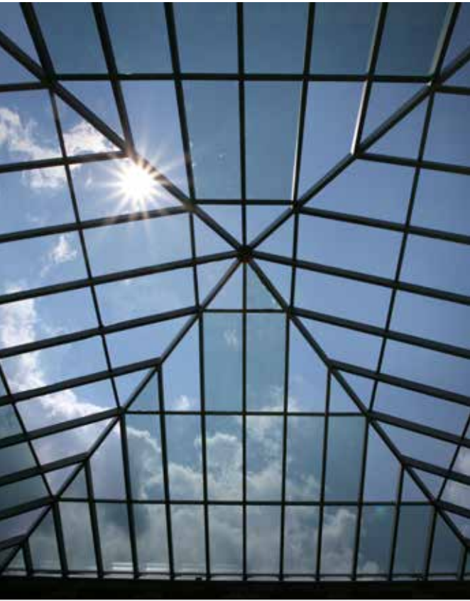
PA ACADEMY OF MUSIC | LANCASTER, PA Irregular Pyramid Skylight
