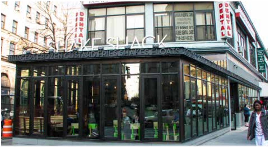
SHAKE SHACK | BROOKLYN, NY Straight Eave Lean-To Sunroom
