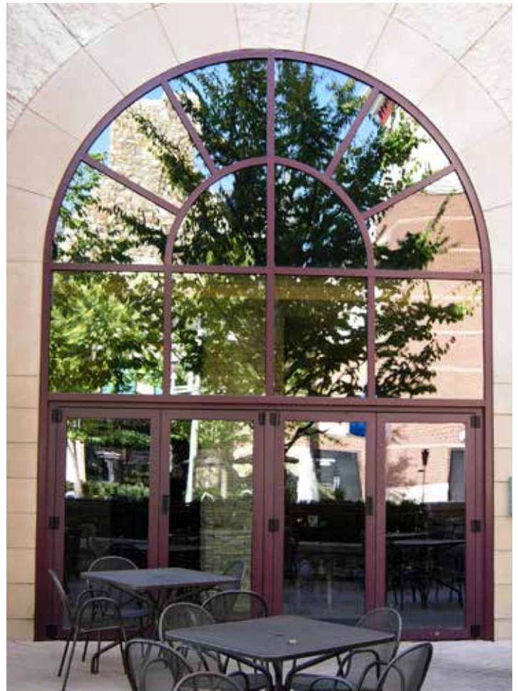
CANTINA COVE RESTAURANT | MANASSAS, VA Aluminum Curtain Wall & G2 Folding Glass Walls
