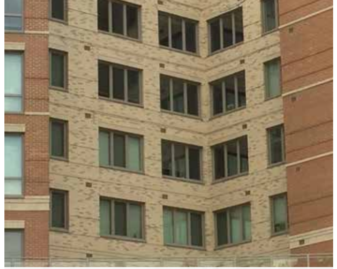
301 WEST BROAD ST APARTMENTS | FALLS CHURCH, VA Vinyl-Composite Terrace Doors, Fixed & Tilt Turn Windows
