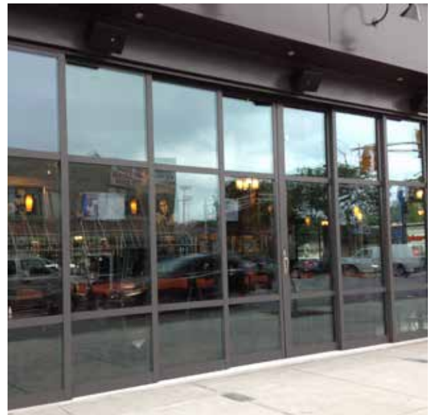
HOPCAT BAR & RESTAURANT | SYRACUSE, NY G3 Multi-Track Sliding Glass Doors
