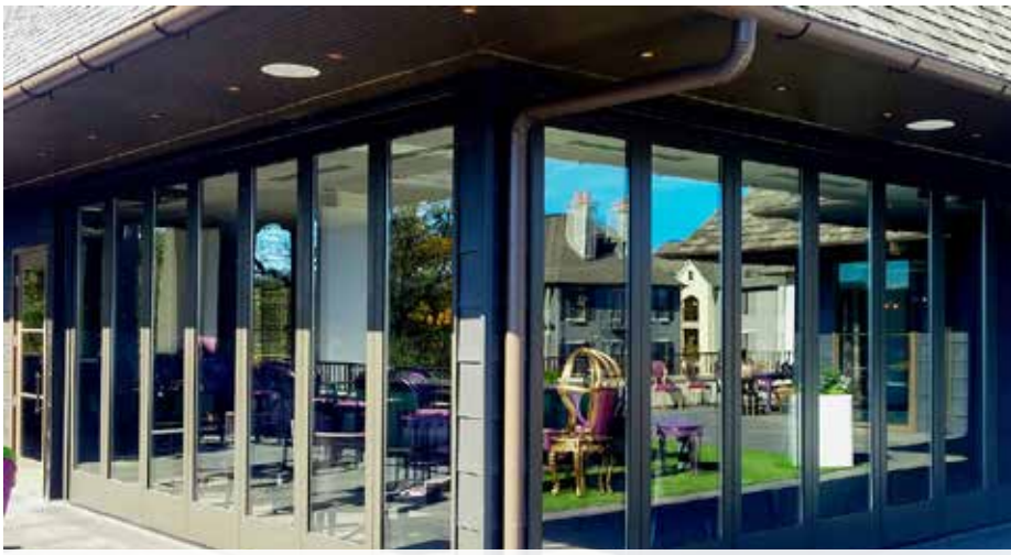
GRAND BOHEMIAN HOTEL | BIRMINGHAM, AL G2 Slide & Stack Glass Walls
