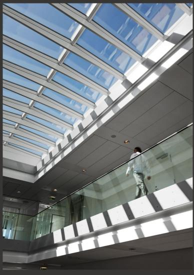
ATP, Vordingborg, Denmark. Ridgelight at  $5\,^\circ$  with Beams, 26 modules.
