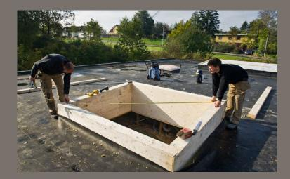
To support an easy installation process, the sub-construction needs to accommodate the very specific system installation. Modular skylights require an accurate fixed-dimension substructure. Likewise, the strength of the sub-construction needs to be calculated from project to project, based on the building design and application size.
