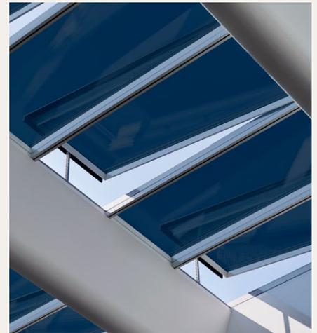
Glazing with electrochrome glass in fully tinted state.
