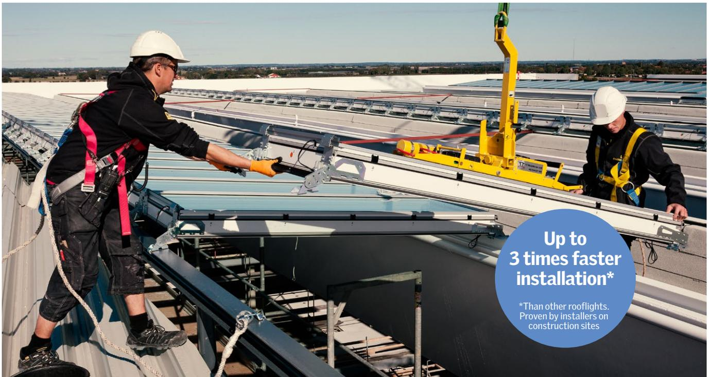
Shielding a building means protecting it against the dangers of weather, as well as, allowing work to commence inside the building. This makes speed a pivotal demand. Modular skylights support the fastest imaginable installation process, starting from delivery on the construction site to fastening the final screw.
