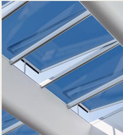
Glazing with electrochrome glass in intermediate state.
