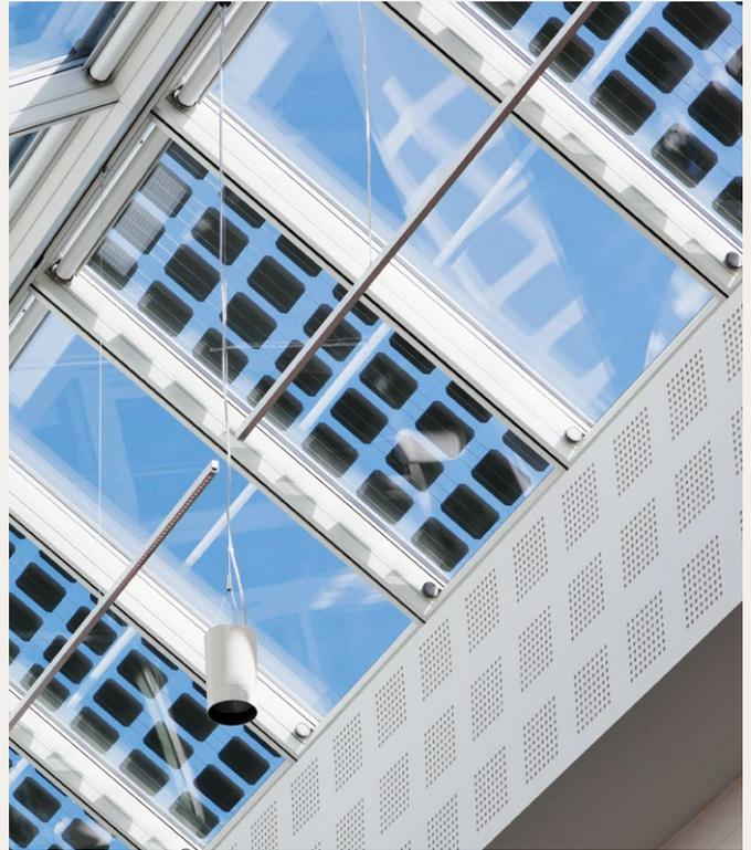
Modular skylights are available with two different types of integrated monocrystalline photovoltaics:
