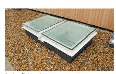
Dual rooflight with drainage gutter
