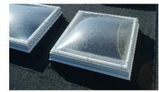
Dome Rooflight with diffused polycarbonate glazing
