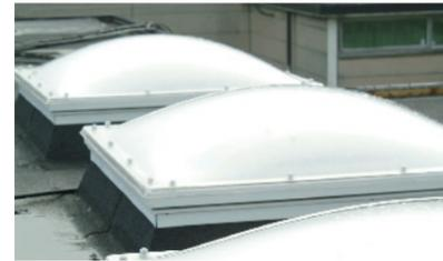
Dome Rooflight with opal polycarbonate glazing
