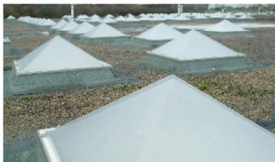
Pyramid Rooflight with opal polycarbonate glazing
