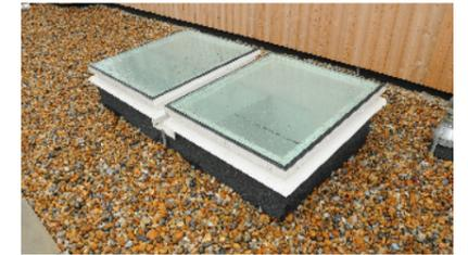
Dual rooflight with drainage gutter
