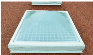
Dome Rooflight with security intruder grid
