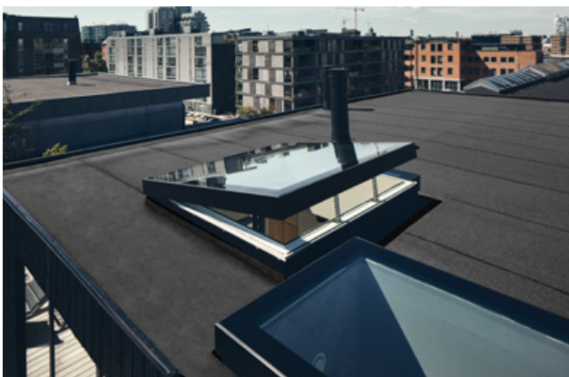
Connecting the electricity and checking the functionality
