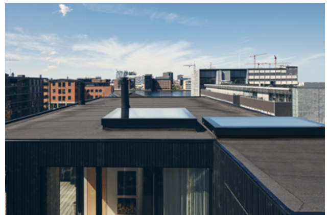
External work finalized
