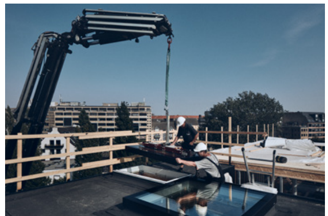
Placing the top unit
