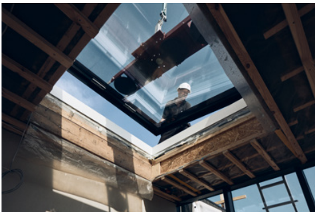
Placing the top unit
