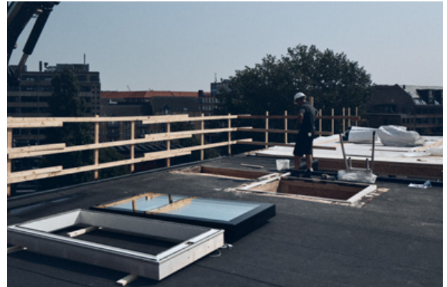
Preparing the hole for the upstand
