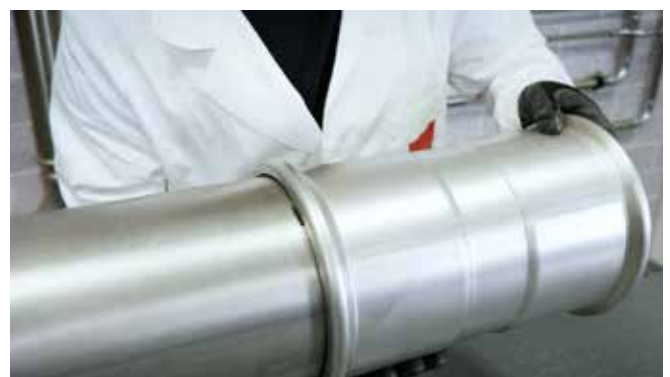
Figure 17 - Inserting pipe into the press fitting
