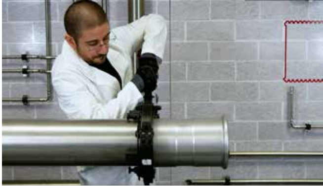
Figure 18 - Making the press connection n° 1
