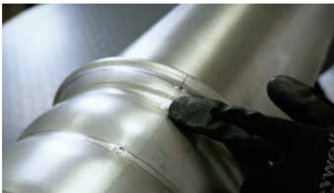
Figure 20 - Checking the press connection
