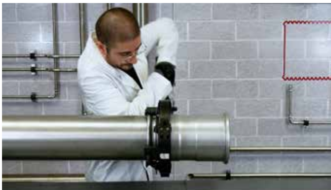
Figure 19 - Making the press connection n° 2
