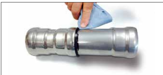
Figure 8 - Cleaning of the grease residual
