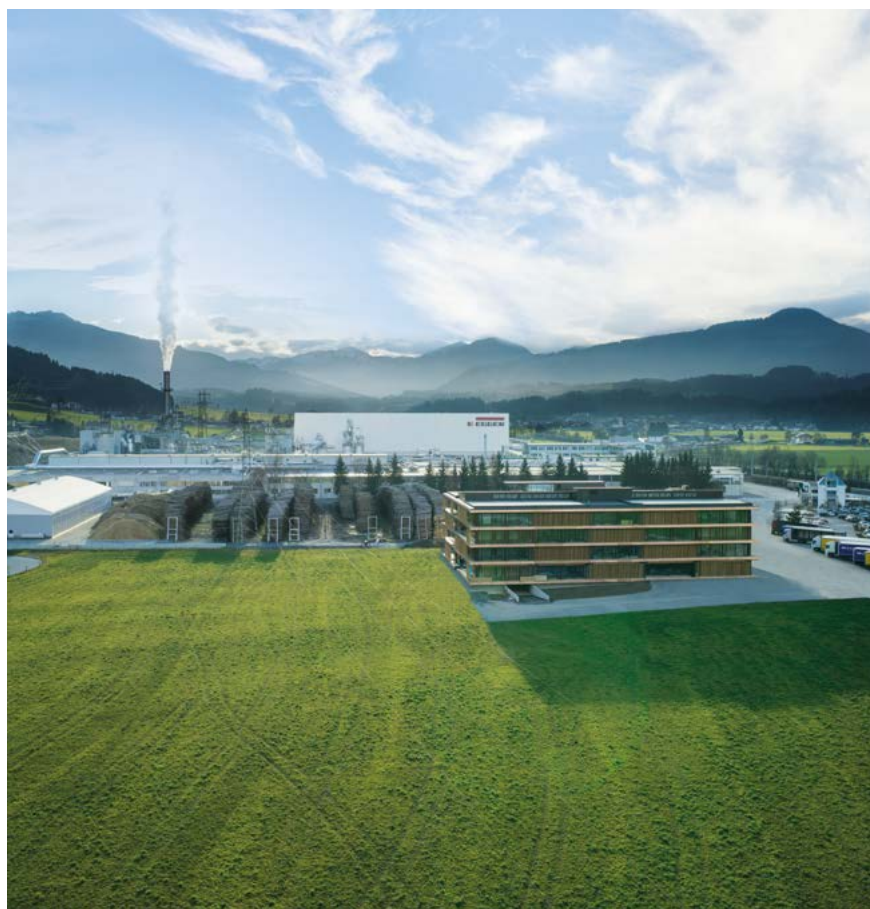
Plant St. Johann Usine de St. Johann
