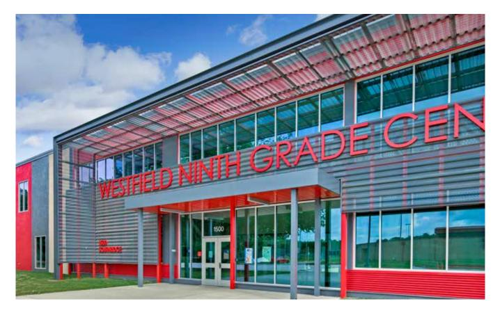
Petersen offers a complete line of exposed fastener panels, allowing for creative design flexibility in a cost-effective yet architecturally attractive metal panel. The versatile 7.2 panel, R-36 and 1/2" Corrugated panels can be specified for a wide range of building envelope applications including roofs, walls and linear panels. The M-36, M-42 and 1/2" Corrugated panels are suitable for wall and equipment screen projects.
