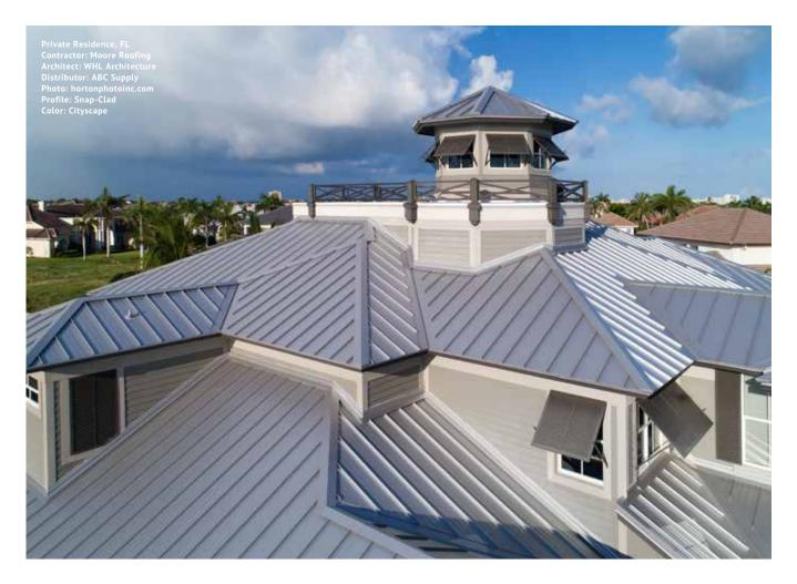
PAC-150 standing seam metal roofing panels combine semistructural metal panel performance with architectural roofing panel aesthetics. PAC-150 roofing coil for field-forming operations is leveled to provide superior panel flatness. Maximum panel length is limited when factory or shop-formed but virtually unlimited when field-formed; minimum panel length is approximately 4'.
