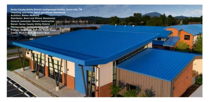
Tite-Loc panels combine structural panel performance with architectural panel aesthetics. Tite-Loc panels are leveled to provide superior panel flatness. A factory-applied sealant bead can be applied for additional weather resistance. Maximum panel length is 64' and minimum panel length is 4'. Consult factory for longer lengths.
