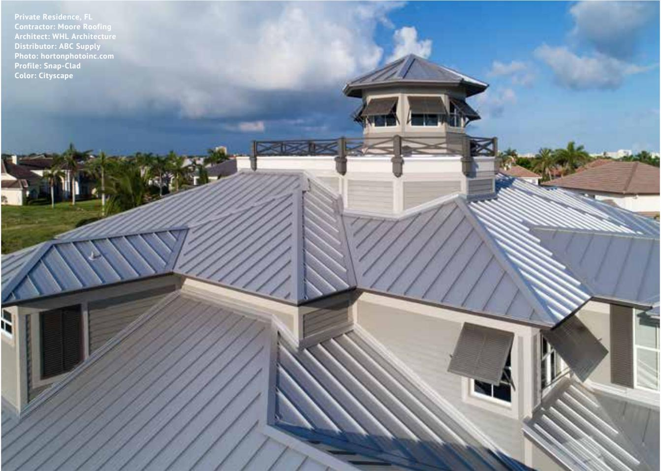
PAC-150 standing seam metal roofing panels combine semi-structural metal panel performance with architectural roofing panel aesthetics. PAC-150 roofing coil for field-forming operations is leveled to provide superior panel flatness. Maximum panel length is limited when factory or shop-formed but virtually unlimited when field-formed; minimum panel length is approximately 4'.
