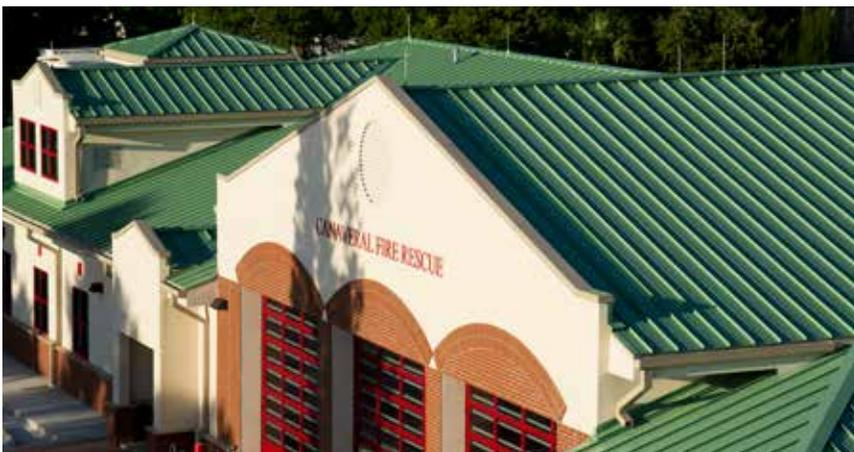
\*24 gauge and 22 gauge steel and .032 and .040 aluminum panels are UL-90 classified over solid substrate. See roof deck construction in Underwriter Laboratories roofing materials and systems directory. \*\*24 gauge and 22 gauge Tite-Loc Plus panels are FM Approved in 12" and 16" widths over 16 gauge open purlins only.
