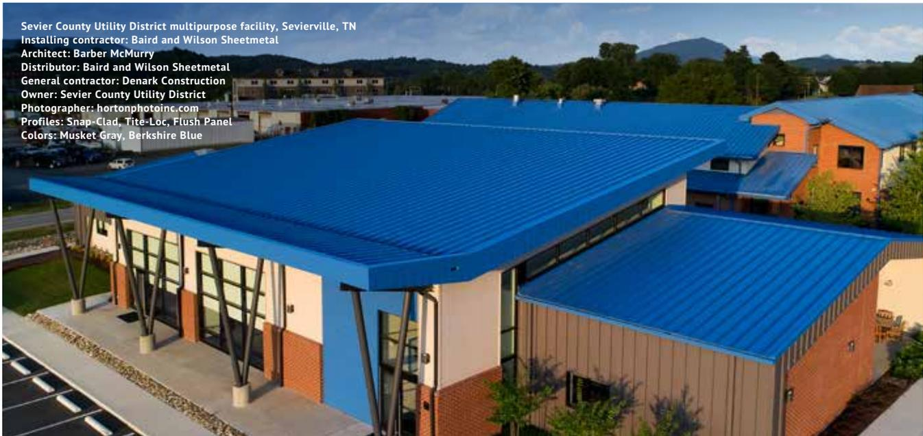
Tite-Loc panels combine structural panel performance with architectural panel aesthetics. Tite-Loc panels are leveled to provide superior panel flatness. A factory-applied sealant bead can be applied for additional weather resistance. Maximum panel length is 64' and minimum panel length is 4'. Consult factory for longer lengths.
