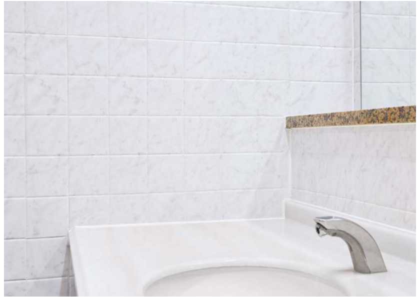
Restroom refurbishment / ST-024TIL
