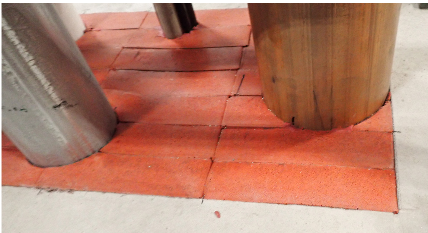
Firestop Block Installation (C-AJ-8338)
