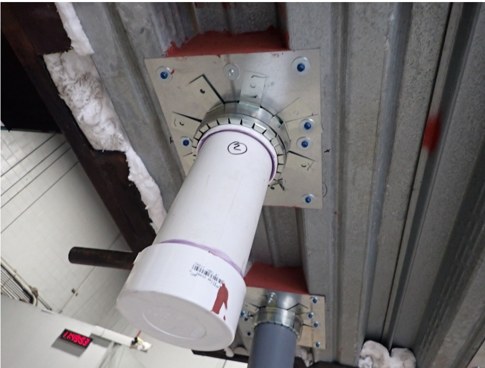
Steel Plate Bridge Across Fluted Deck Allowing Collar Installation (F-A-2419)
