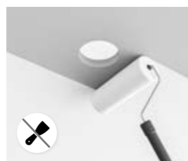
Paint the ceiling, no puttying needed
