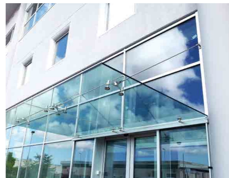
Canopy mounting on the facade uprights (specific accessories). Made by C.i.s.m.e.r. in Aprilia.
