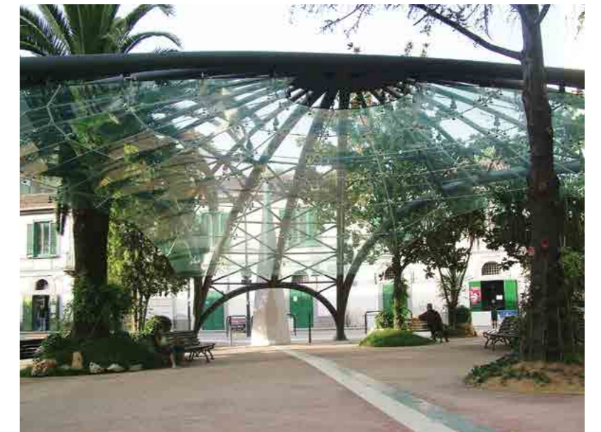
Covered square in Pontecagnano (SA). Place couverte à Pontecagnano (SA).
