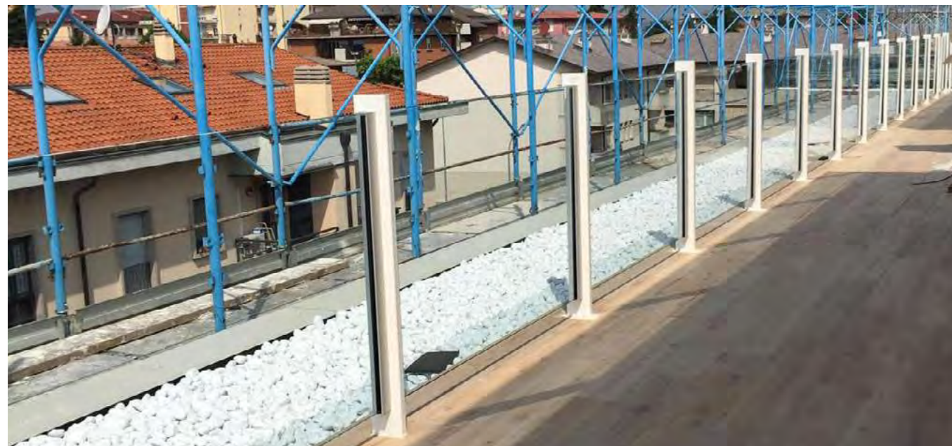
Terrace with Giulietta system completed
