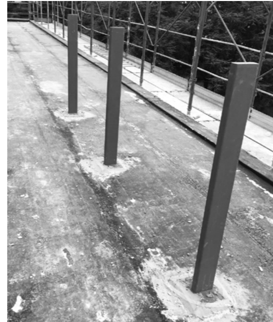
Construction site image before installation of Giulietta
