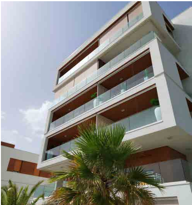
Residential building, Jesolo
