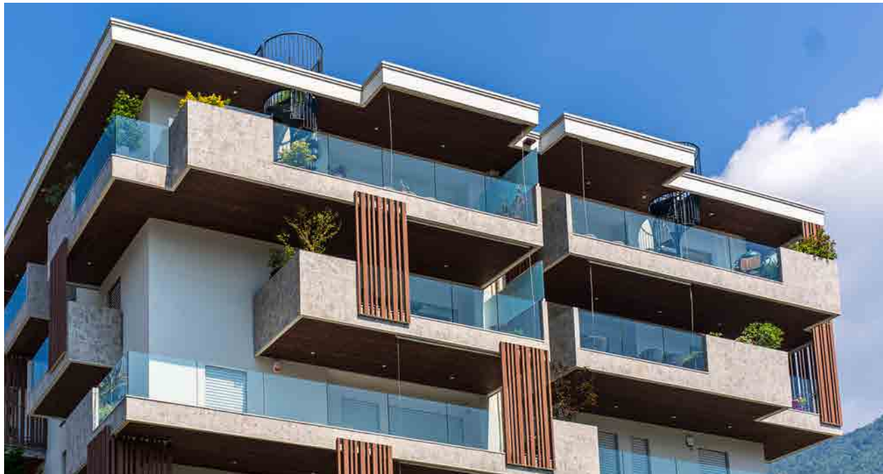
Residential building, Milan
