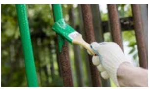
Maintenance with specific antirust treatments for common metal balustrades is recommended, to prevent them from being corroded by time, losing beauty and safety.
