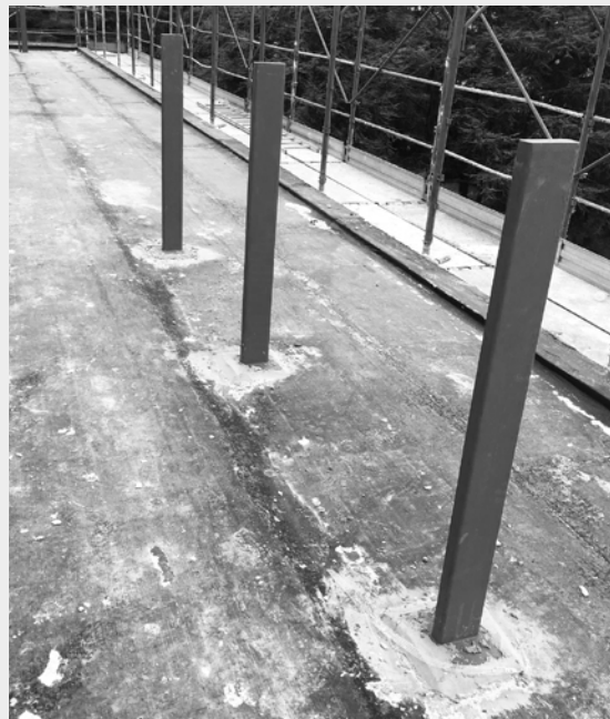
Construction site image before installation of Giulietta
