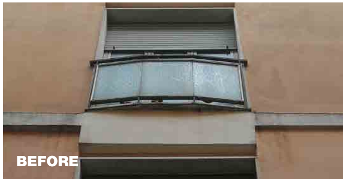
Example of a building with non-standard French balconies with wired glass.
