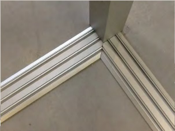
Mitered bottom track next to 4x4 vertical post.
