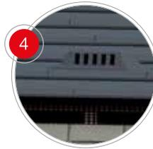
Ventilation roof tiles are installed in the same manner as other roof tiles, interlocking into each other laterally and from the top. These roof tiles should be distributed along the roof surface.
