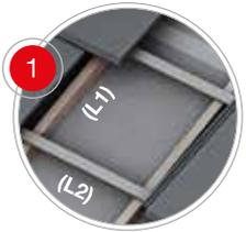
A breathable waterproof membrane should be laid on the support of the roof and the main battens (L1) should be installed every 50/70 cm, parallel to the steepest slope. The horizontal support battens (L2) for the roof tiles should be fixed to the main battens depending on the useful length of each roof tile (the useful length must be calculated on site).
