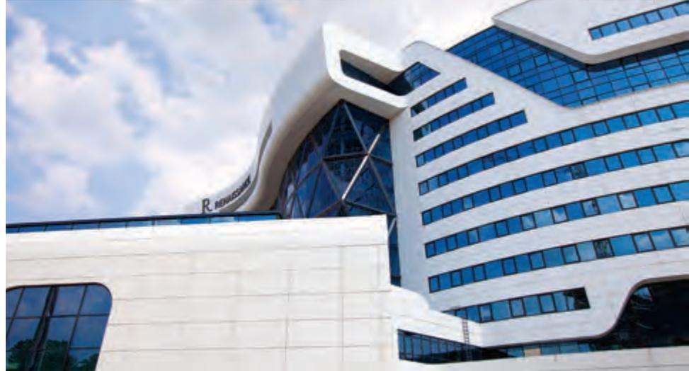
System is intended for cladding of facade blocks fastened to reinforced concrete slabs what is the one safe foundation.
