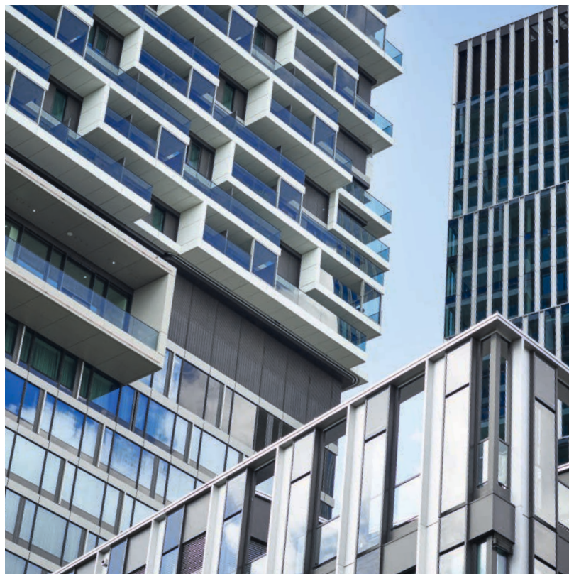
One Forty West, Frankfurt am Main, LEED – Core and Shell certified IGP-DURA ® xal 42, photo and cover image by Alexander Bernhard
