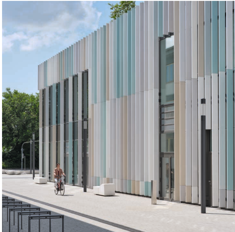
InformatiKOM institute building, Karlsruhe — IGP-HWFclassic 59 Photos by Swen Carlin
