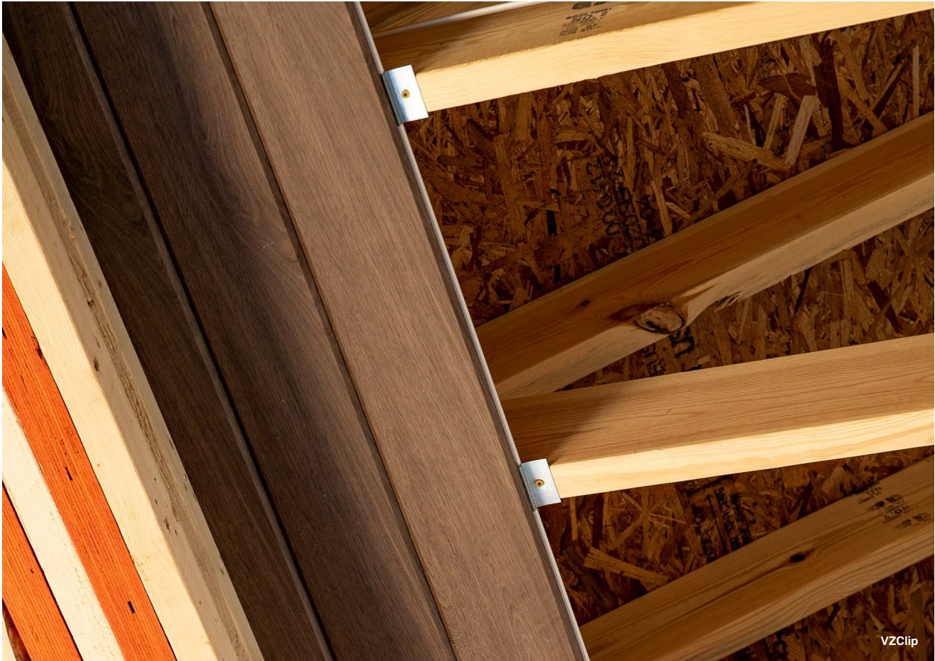
XCEED Siding Nail Hem Bracket
