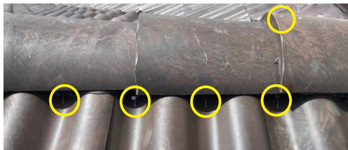
Figure 2.7.5 Exposed Fasteners
