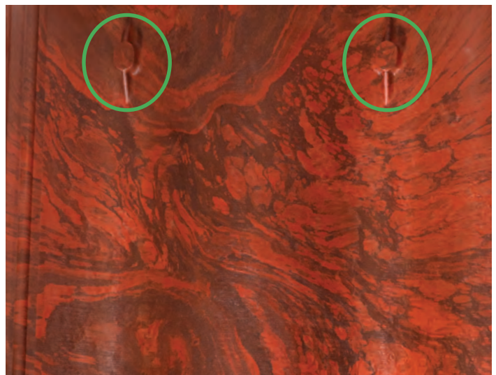
Figure 2.7.3 Fastener locators (front)
