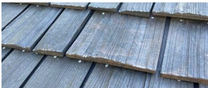
Figure 2.7.6 Exposed Fasteners
