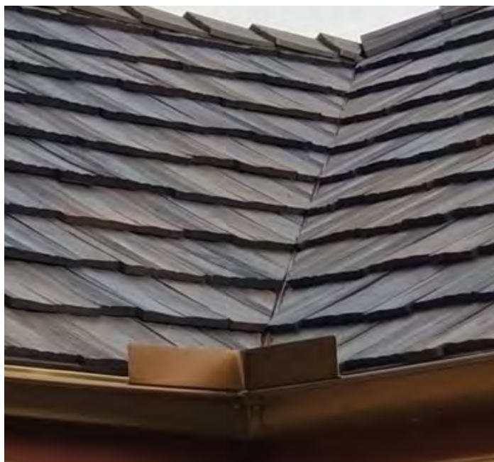
Figure 3.6.7 Closed valley example with 1 ½" center crimp
