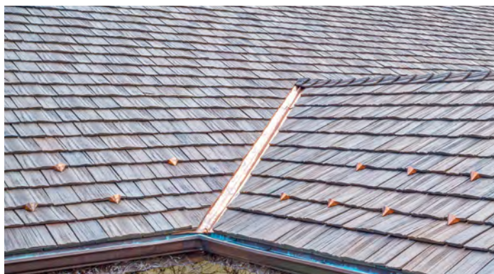
Figure 3.6.6 Open Valley Example with minimum 1" center crimp
