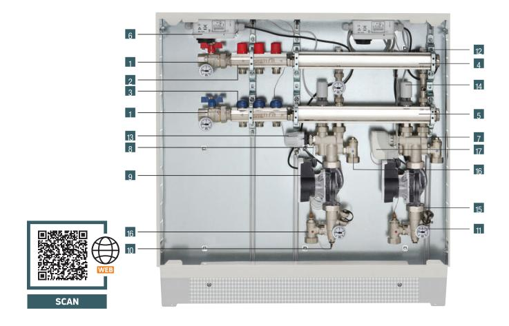
The distribution system allows for the construction of systems with high temperature zones (radiators, fan coils) and low temperature zones (underfloor systems).
