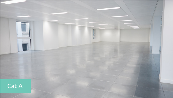
A landlord-fitted space with standard ceilings and services, typically using basic grid systems, functional but with minimal acoustics.
