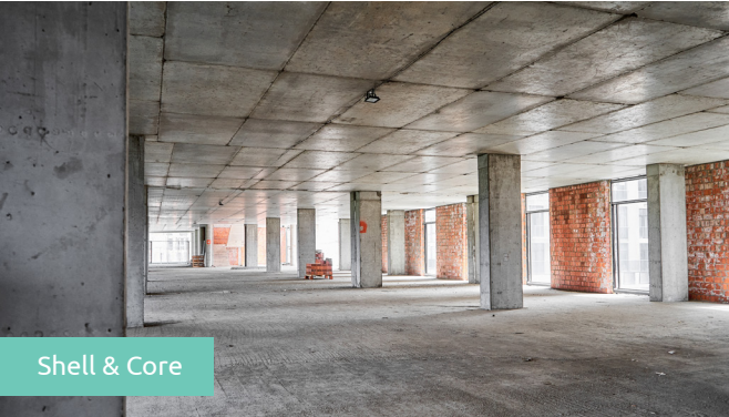
The base building with no internal finishes or ceilings, typically an exposed soffit. It offers maximum flexibility but no acoustic performance.
