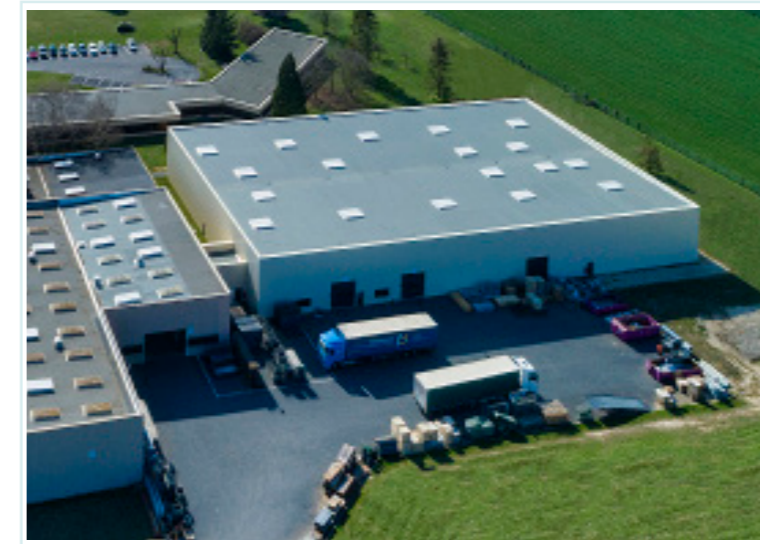
Logistics department, new building with 3 000 sqm - Activity fully integrated to OB Profils -
