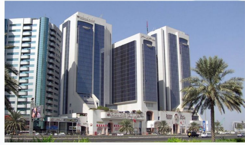
Crowne Plaza (Renovation Project) , Dubai
