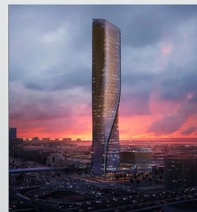
Wasl Tower, UAE
