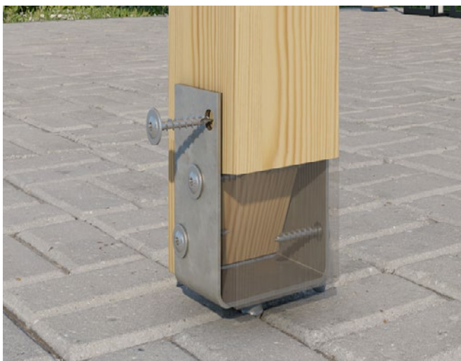
Joint between post base and post
