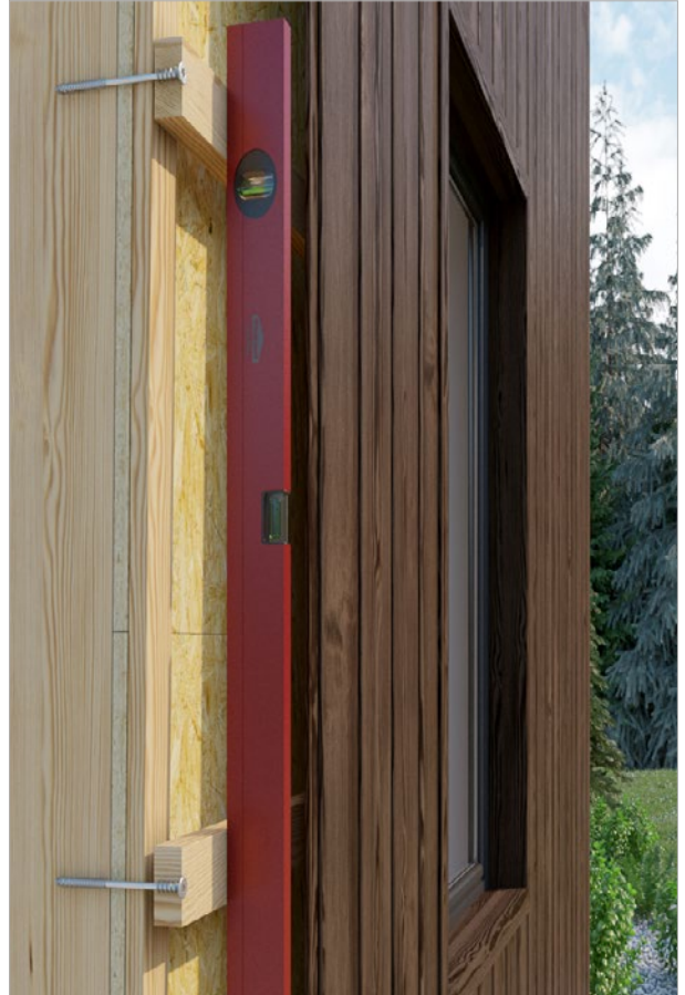
Levelling of facade substructure
