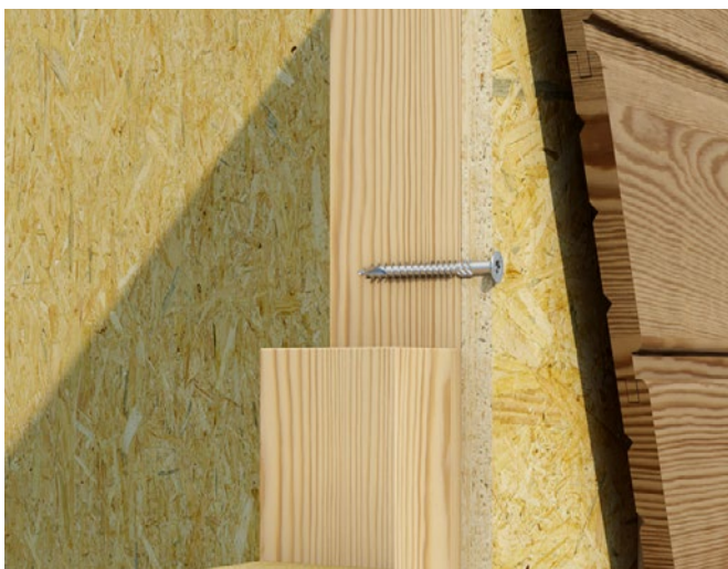
Fixing boards to wooden structure in facade construction
