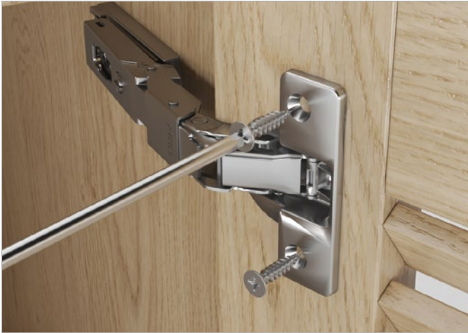
Installation of hinges
