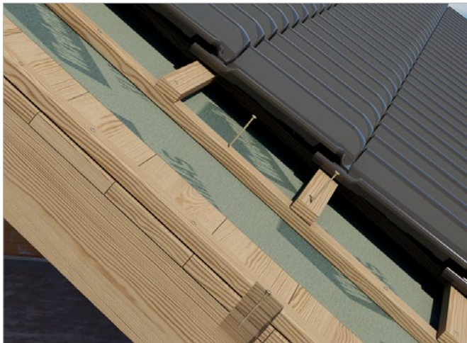
Fixing of battens and counter battens
