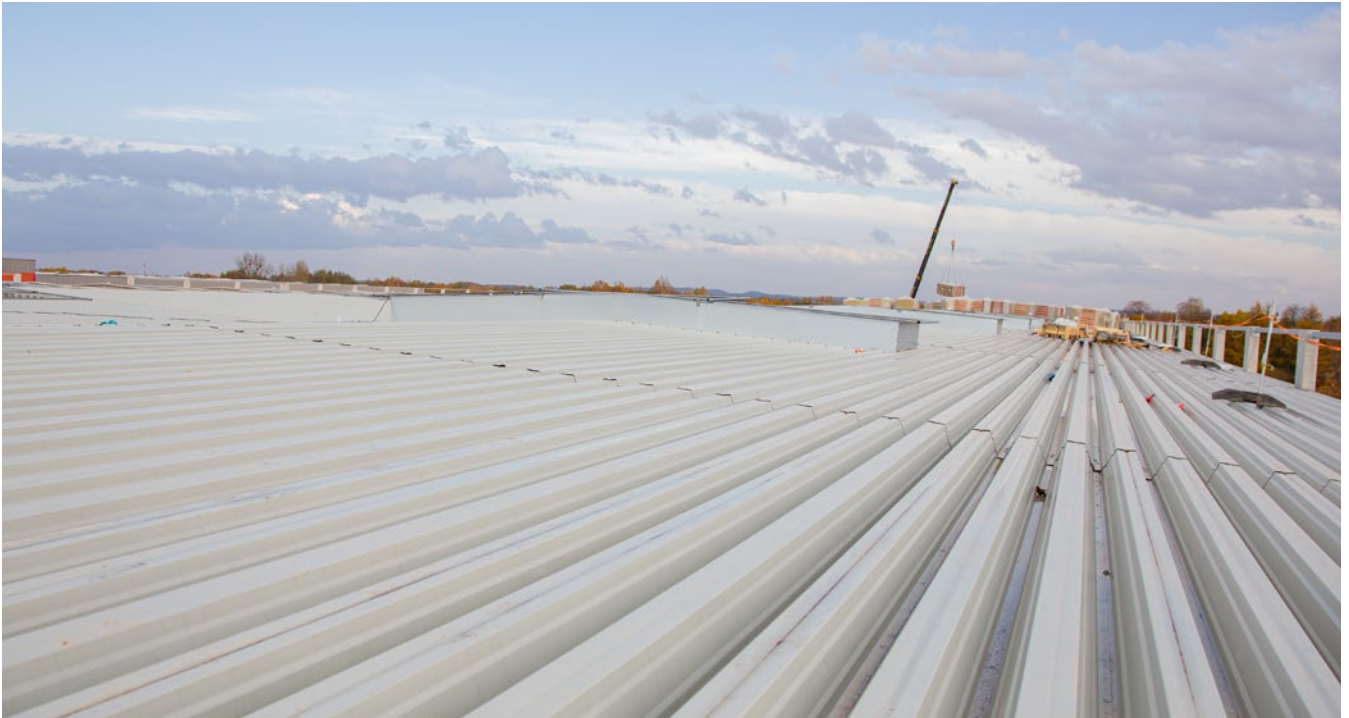
Longitudinal fastening steel sheet profile
