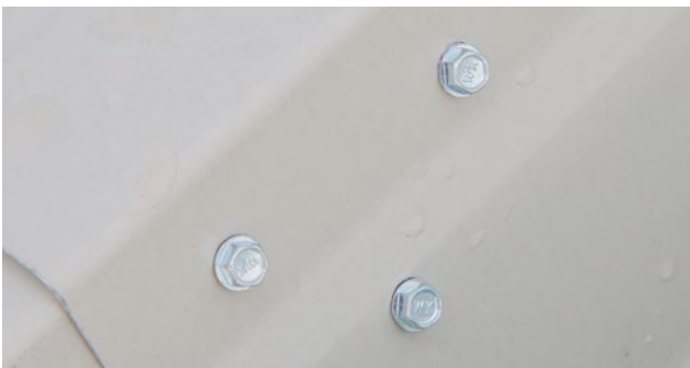
Longitudinal fastening steel sheet profile
