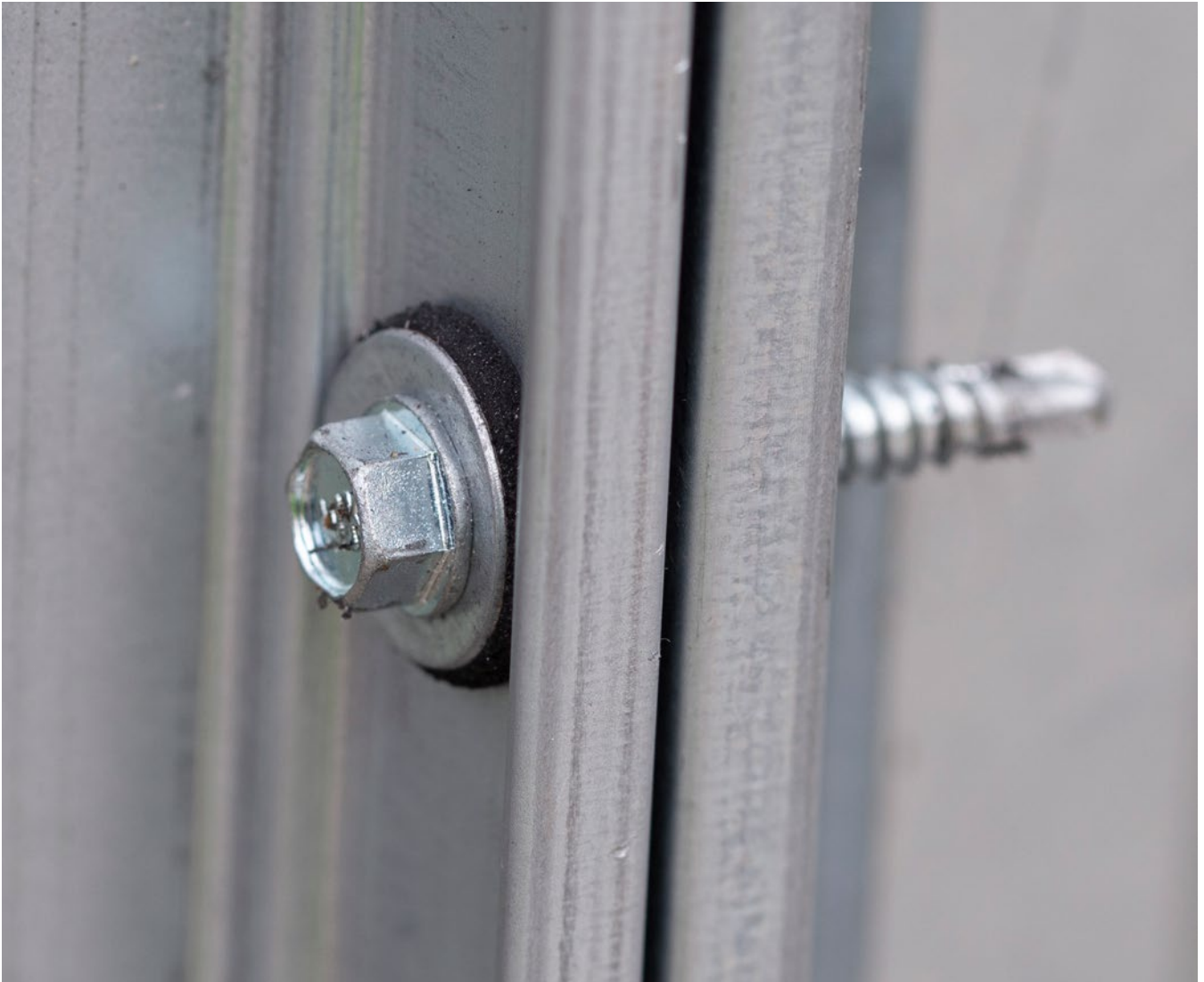
Fastening two layers of steel sheet profile
