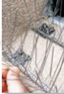
Glue Clip Installation
