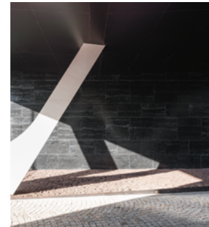
▲ The Travertin concrete pattern is combined with black concrete for an especially high-end finish.
