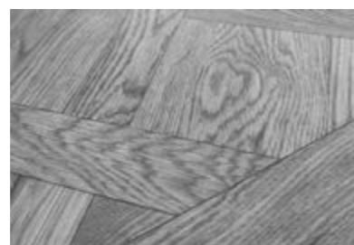
Versailles wood structure *
