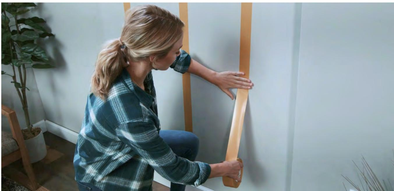
**Step 2:** Starting from where the lowest row will be, apply adhesive between the tape, using just enough to add Audimute Strata pieces before the adhesive dries.
