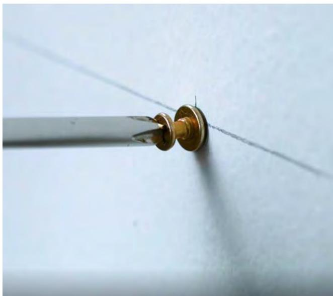
**Step 5:** Hang the panel by sliding the keyhole plates over the double headed screws in the wall.
