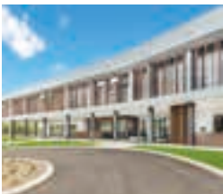
Fujitsu General (Aust.) Pty Ltd. (Australia)
