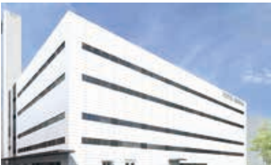
Technology research building (Japan)
