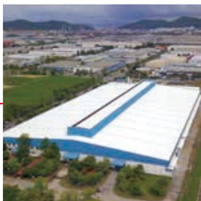
Fujitsu General (Thailand) Co., Ltd. (Thailand) Factory-2
