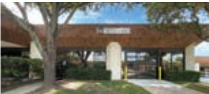
North America R&D Center (USA)
