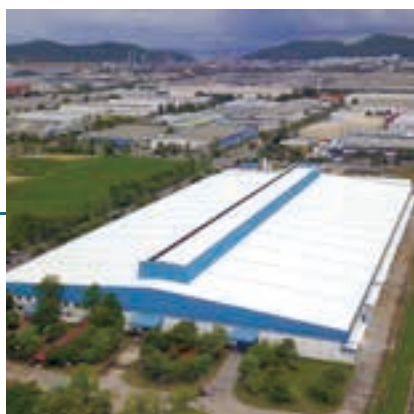
Fujitsu General (Thailand) Co., Ltd. (Thailand) Factory-2
