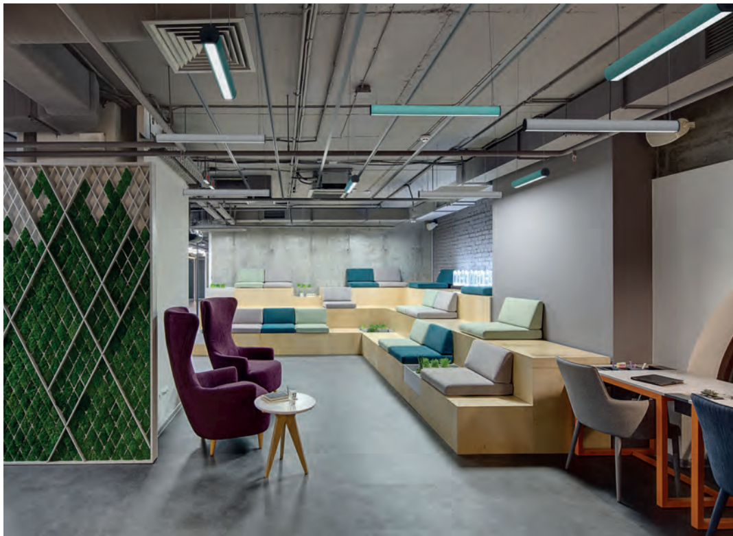
Spaces with visible installations (without false ceiling).
