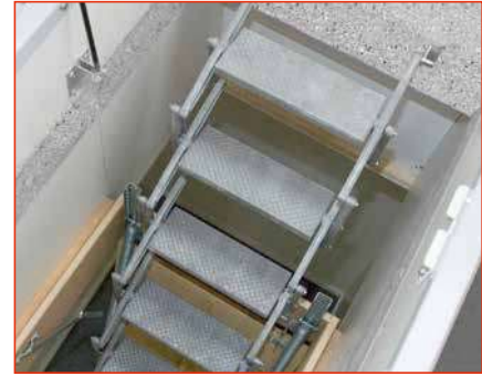
» Extension of scissor stairs (plenum 3)
