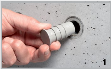
Position and drive in the STOPPER mini
