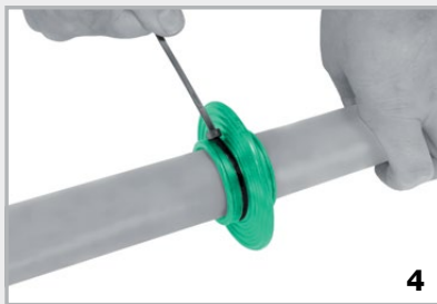
Tighten both fastening straps by hand
