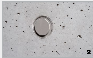
Sealing of distance tube with lip
