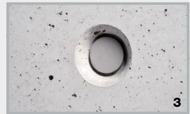
Sealing of distance tube with cone
