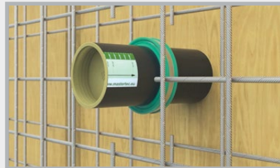
The wall sleeve is attached to the formwork.
