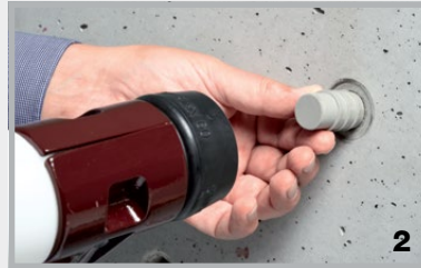
The STOPPER in is driven in with a 1500-2000 g hard rubber mallet.
