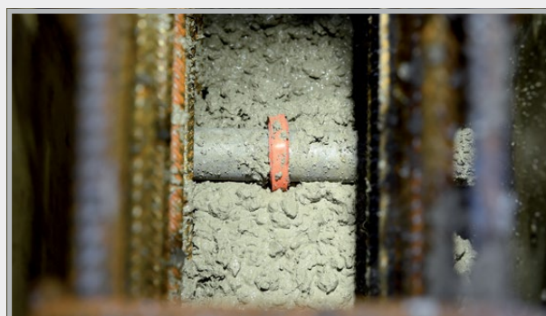
At the construction site
