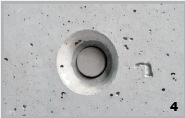
Flush seal for distance tubes with cone.
